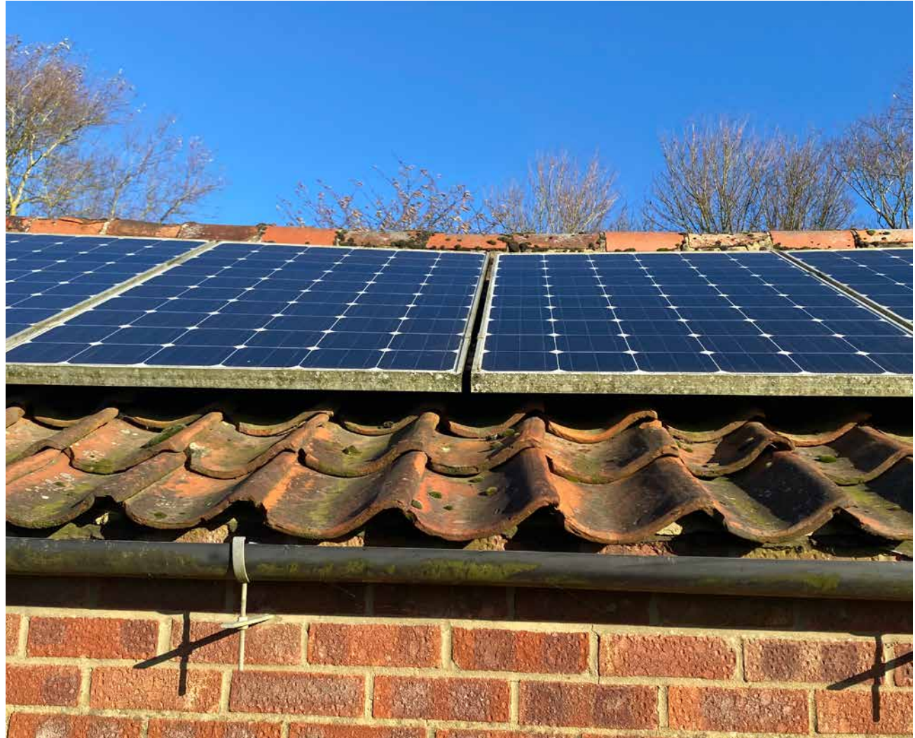
Figure 33: Example of solar panels that have been fitted to an existing building in Sporle with Palgrave.
