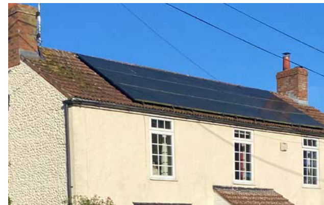
Figure 20: Image of cream render house with solar panels on the roof.
