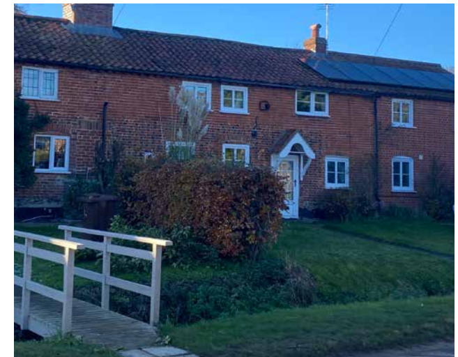
Figure 15: Example of typical terrace farm cottages with characterful front gardens.
